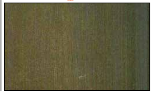
After RUSTRESOLVE Application
